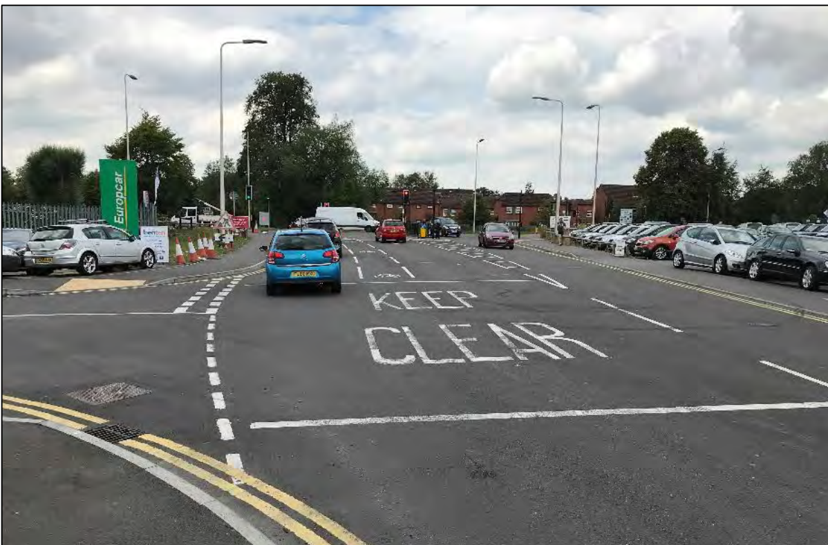
Figure 2 – View of Fleming Road Towards the A339 All Moves Signalised Junction
